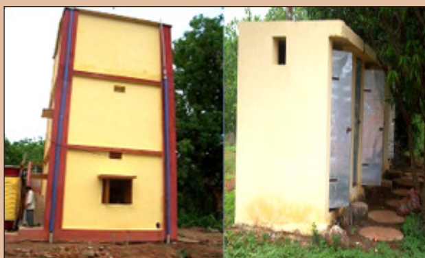
Water supply tank (left) and a toilet-bathroom unit (right)
